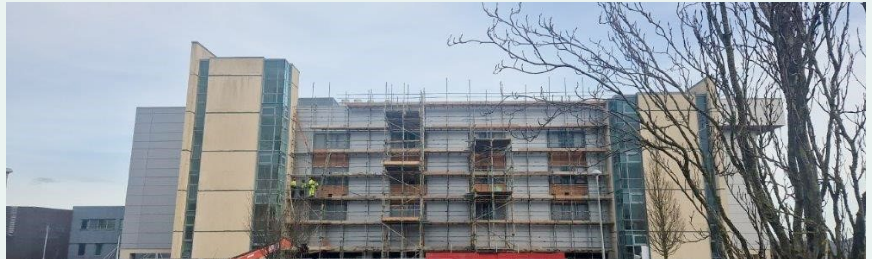
Above: Cardiac Renal Centre Refurbishment.
